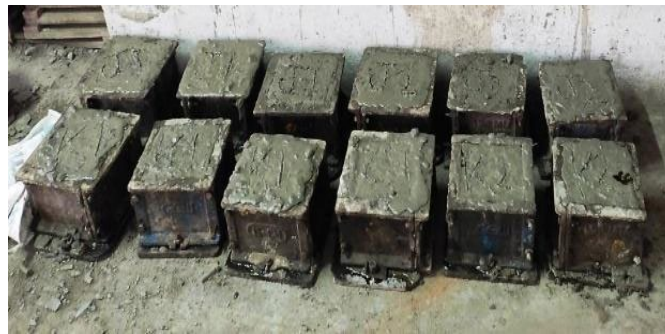
Figure 5 Casting of concrete cubes
