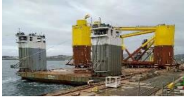
Figure 7 Load-out HTV (Credit Principle Power)
