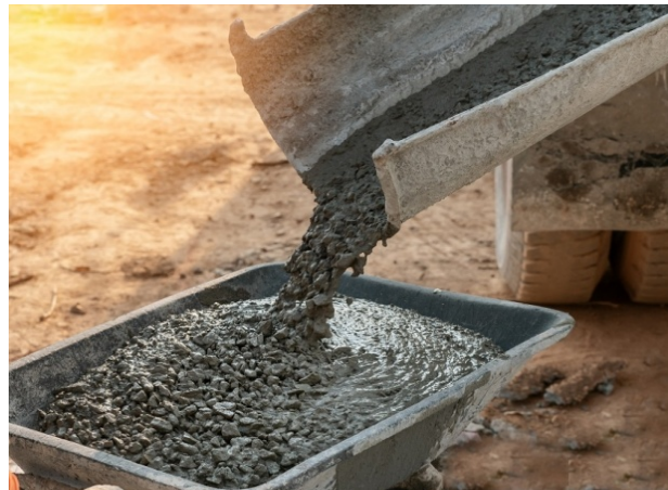
Figure 2: Cement and concrete work
