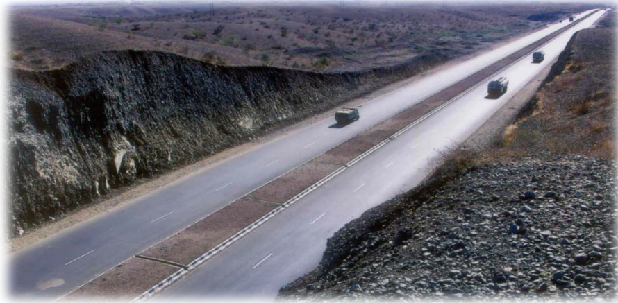
Figure 1: strengthening and widening of (Bagodara –Rajkot) road project
