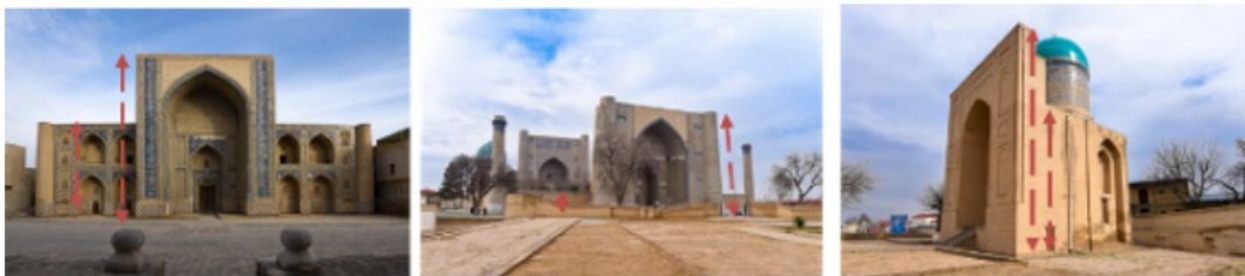
Figure 22: Contrast in Timurid's Architecture Facades, Source: architectureofcities.com
