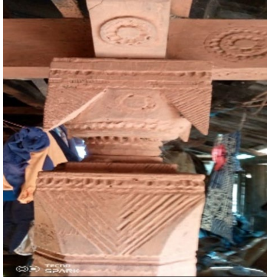
Figure 7 The wooden pillar is noticed at Guma village of Kutia Kandha Community, Belghar, Kandhamal district.
